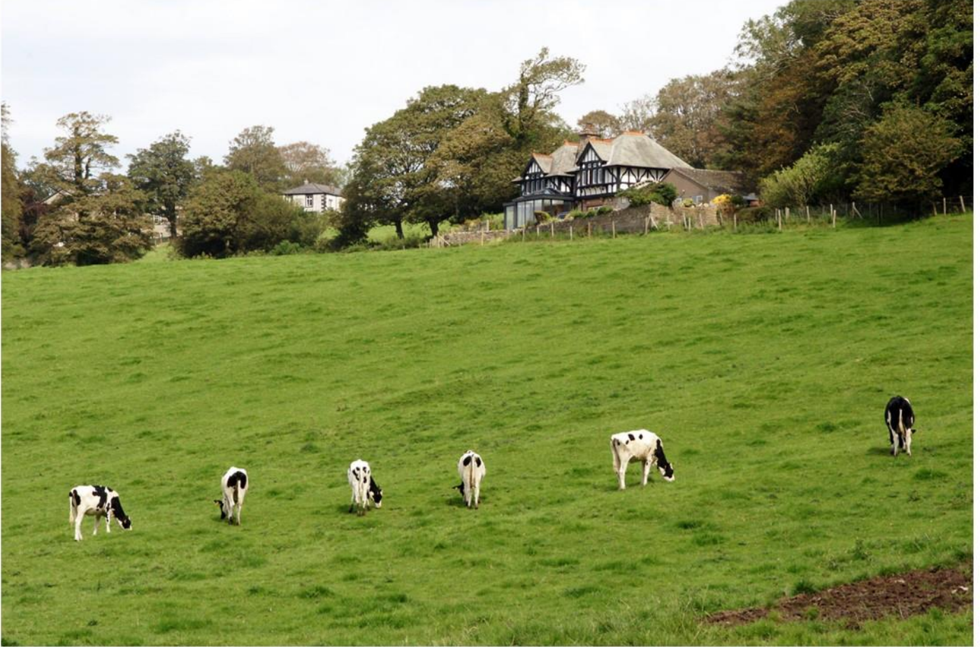
'Walnut Bank Lodge' Stodday pioneering 'shuttered concrete' construction
