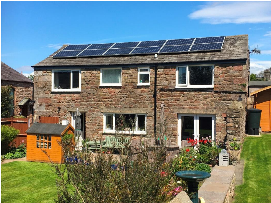
Solar panels on a house in Aldcliffe
